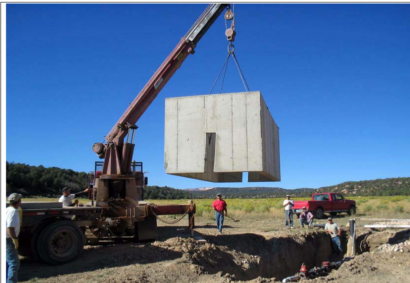
Installing the vault at the new well started out just fine...
